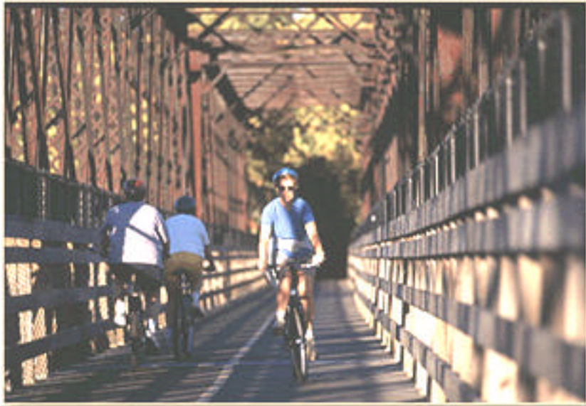
Figure 1. CT River Bridge between Hadley & Northampton Source: http://www.state.ma.us/dem/parks/nwrt.htm
